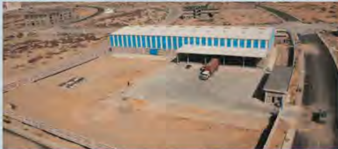
An Aerial view of MAL Pakistan warehouse facility at National Industrial Park, Korangi Industrial Area, an impressive mega structure with over 17000 sq. ft. of warehouse space. MAL Pakistan is one of the first companies to start operations at N.I.P., Karachi.
