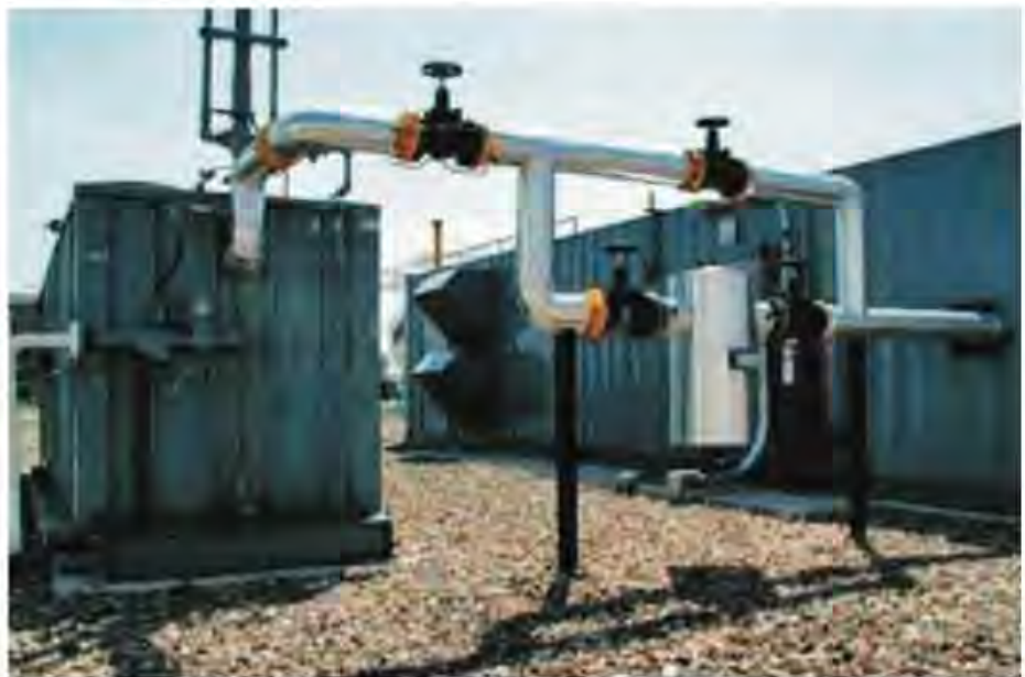
According to officials, comprehensive site surveys have been conducted to select potential points for the establishment of air-mix plants
