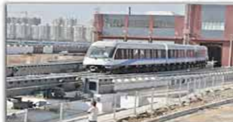
Changsha Express Transit, utilizing electromagnetic levitation technologies.
