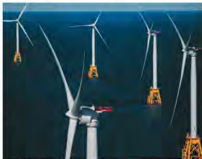
The GE-Alstom Block Island Wind Farm stands in this aerial photograph taken above the water off Block Island, Rhode Island.-Bloomberg
