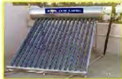
Solar Thermal Geyser
