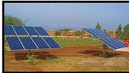
5 KW SOLAR PUMPING SYSTEM - TARNOL RWP
