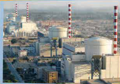
CNPGS Supplying Electricity to National Grid at Highest Capacity Factor
