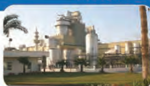
Proctor & Gamble Ariel Plant - PAK
