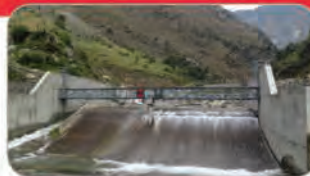
18 MW Ranolia Hydro Power - PAK
