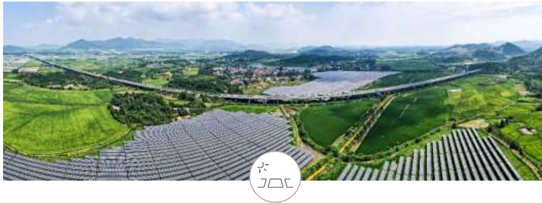
Centralized PV power station
