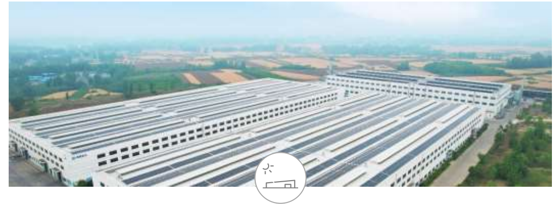
Industrial & commercial PV power station
