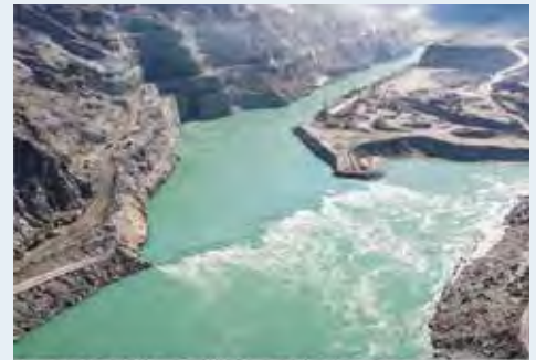
Diامر Basha Dam Project: River Diversion through Test Run
