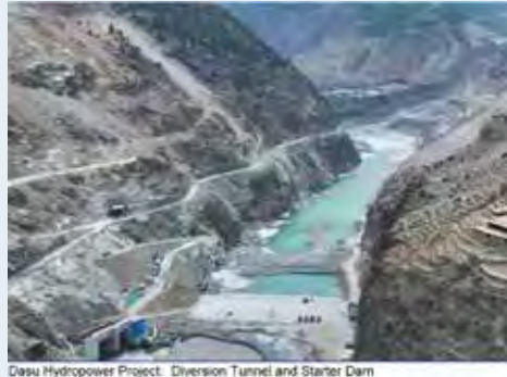
Dasu Hydropower Project: Diversion Tunnel and Starter Dam
